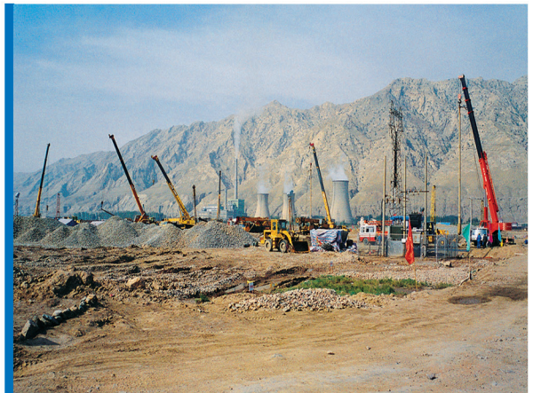
Fundamental vibroflotation project of Inner Mongolia Wulashan Power plant 内蒙古乌拉山电厂基础振冲工程
