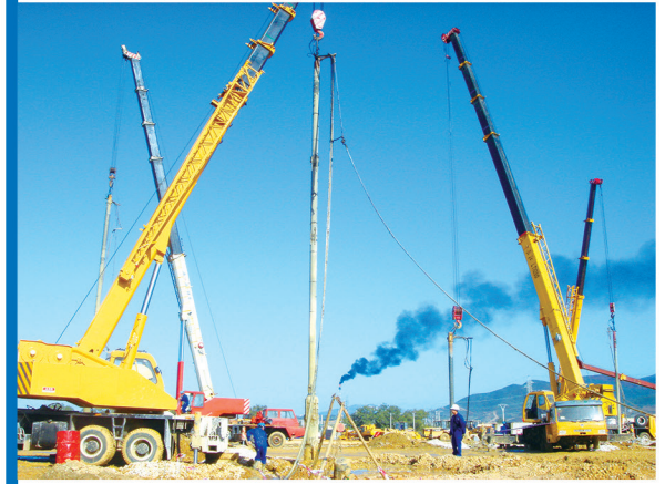
Vibroflot pile for 5million tons annual condensate oil project in Algeria 阿尔利亚 500 万吨年凝析油项目振冲桩
